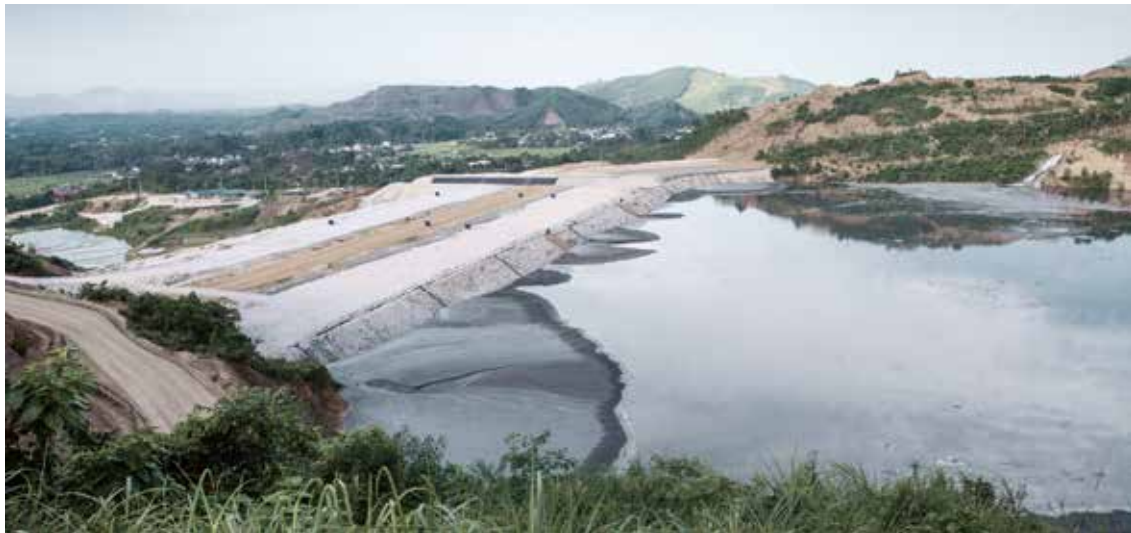
A corner of Tailing Dam
