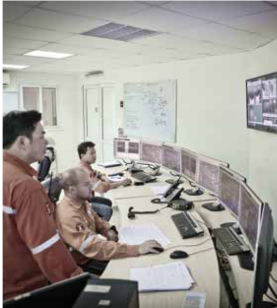
In Control room
