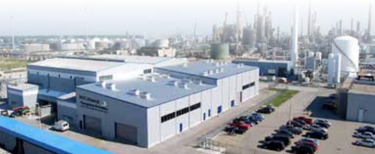
H.C. Starck Canada – Sarnia plant
