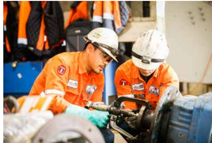
MHT Maintenance engineers working on site (Vietnam)
