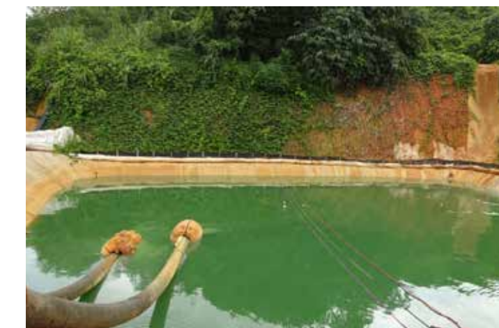
The seepage collection sump from mineralized waste stockpile
