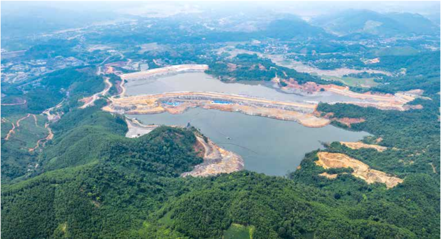
Overview of NPMC tailing dam in Vietnam
