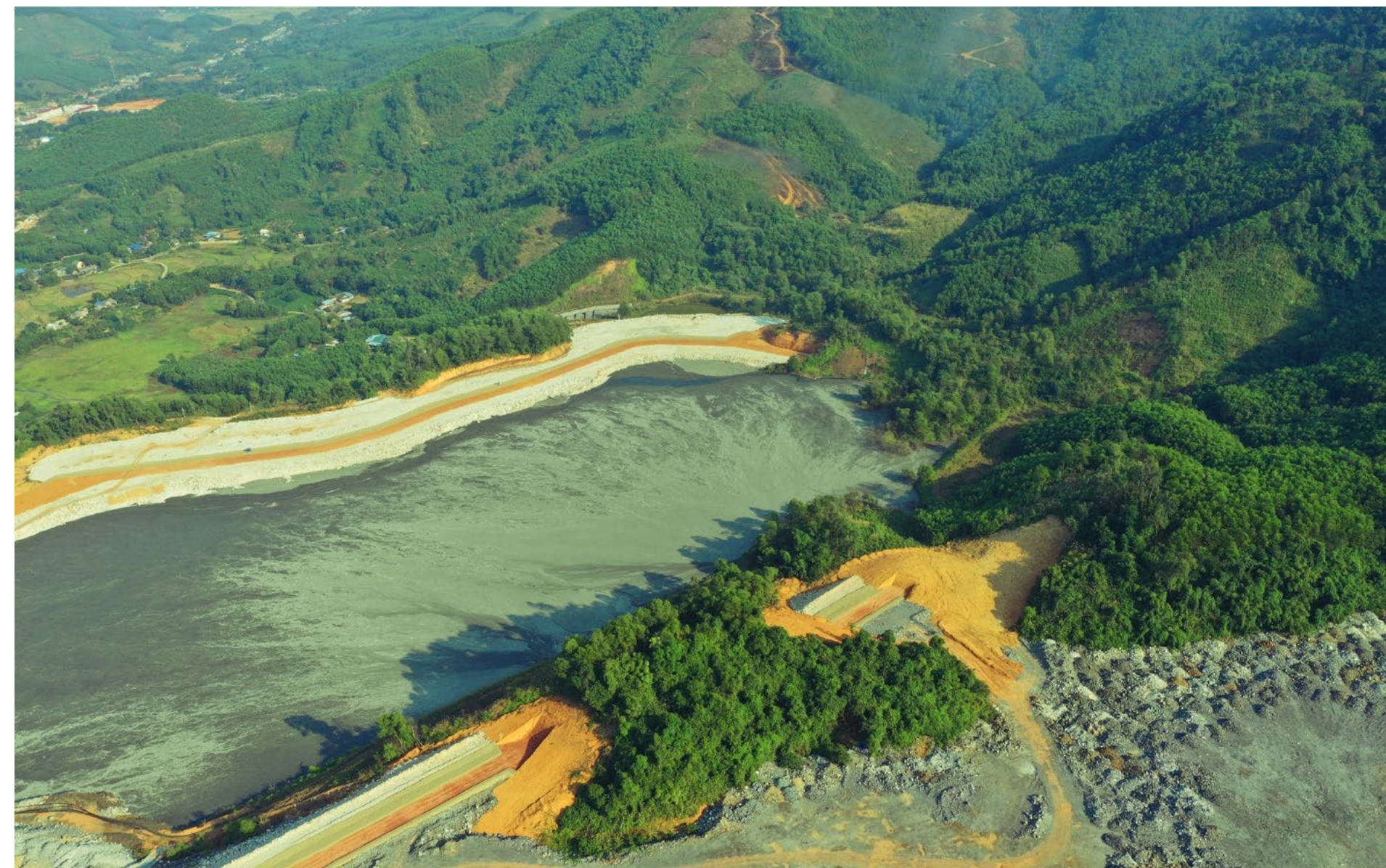
Tailings Dam for recycling
