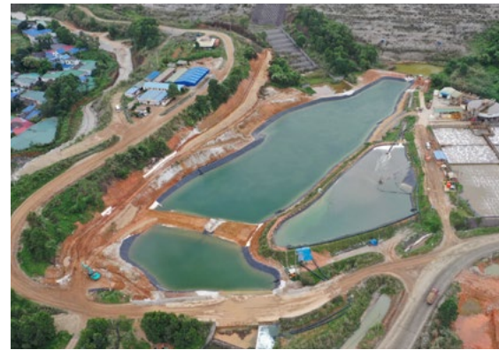
Completed the TSF-SP pond lining
