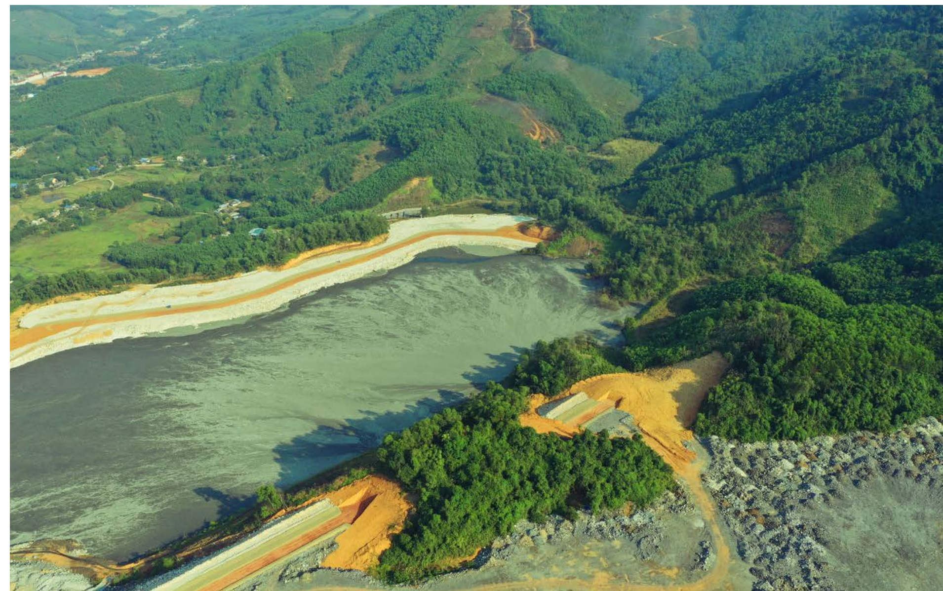
Tailings Dam for recycling
