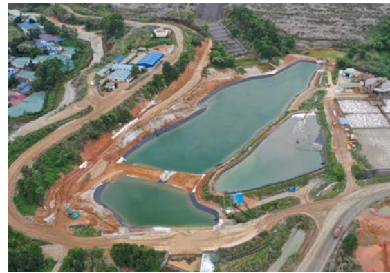
Completed the TSF-SP pond lining
