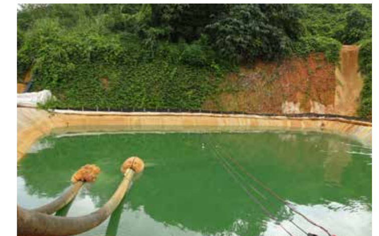
The seepage collection sump from mineralized waste stockpile
