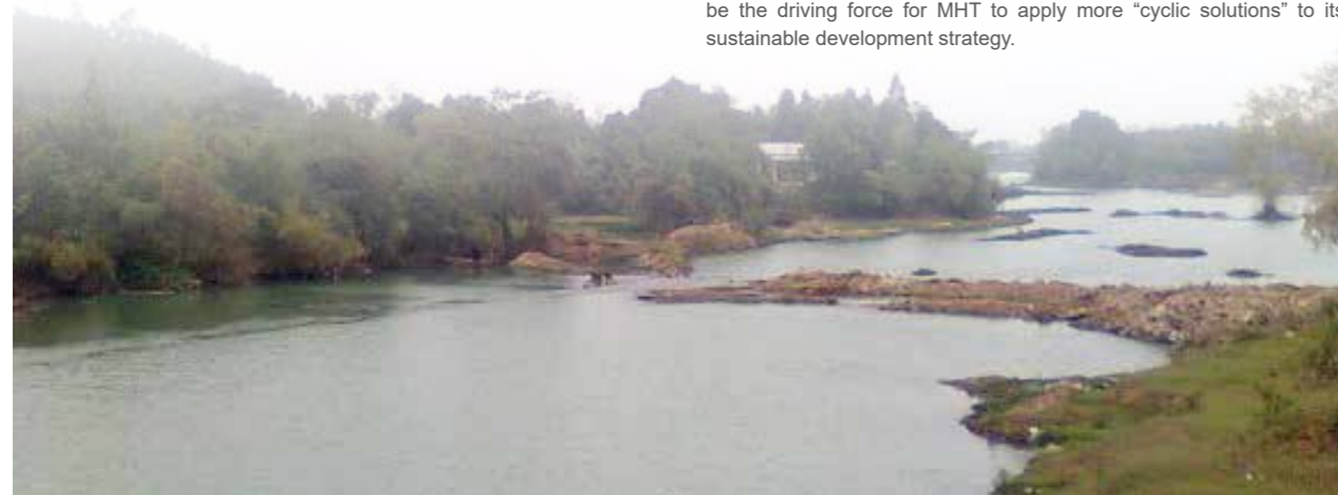
Cong river – water resource supply to NPMC processing plant
