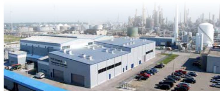
H.C. Starck Canada – Sarnia plant
