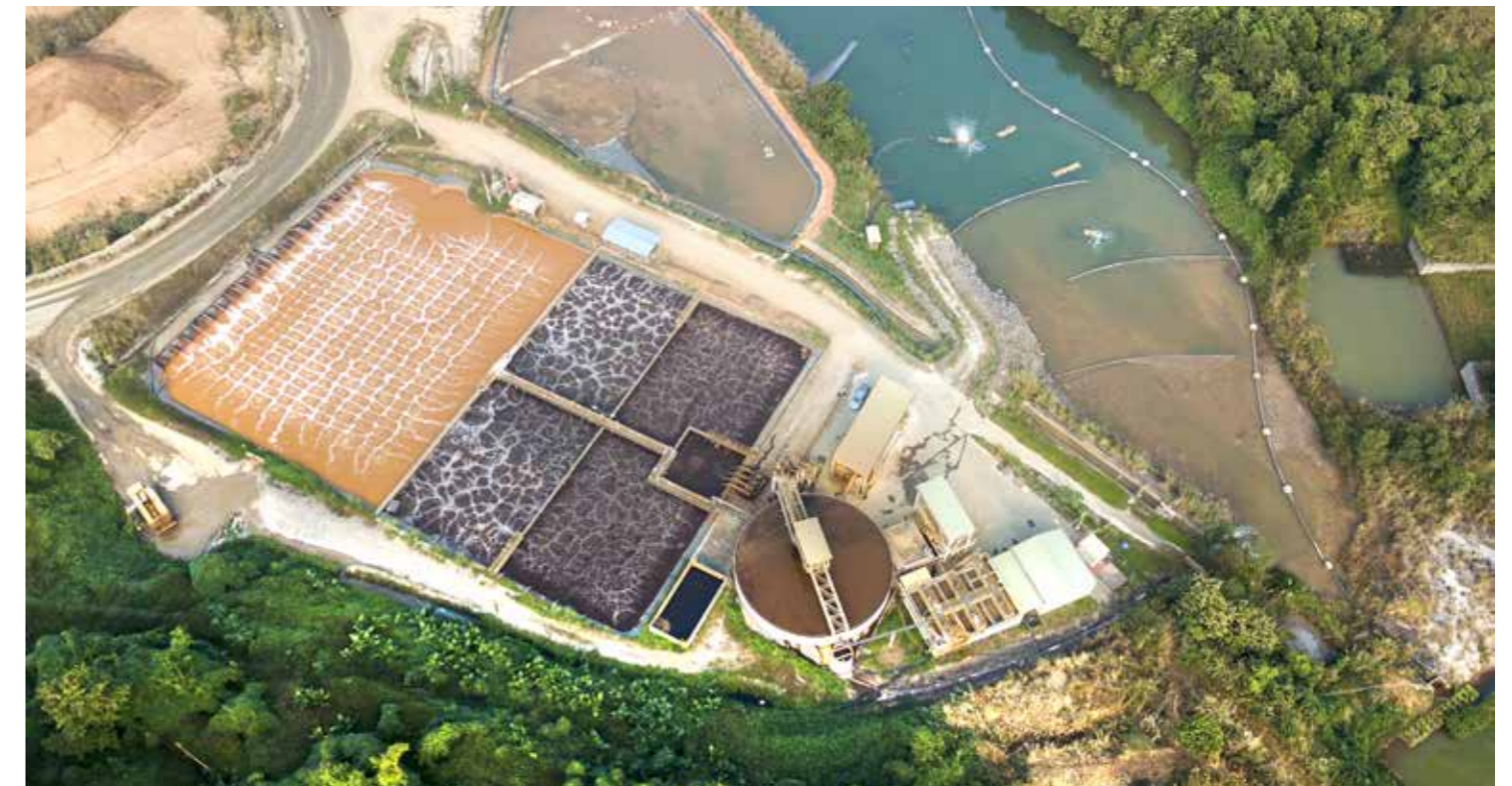
Overview of MHT waste water treatment plant in Vietnam
