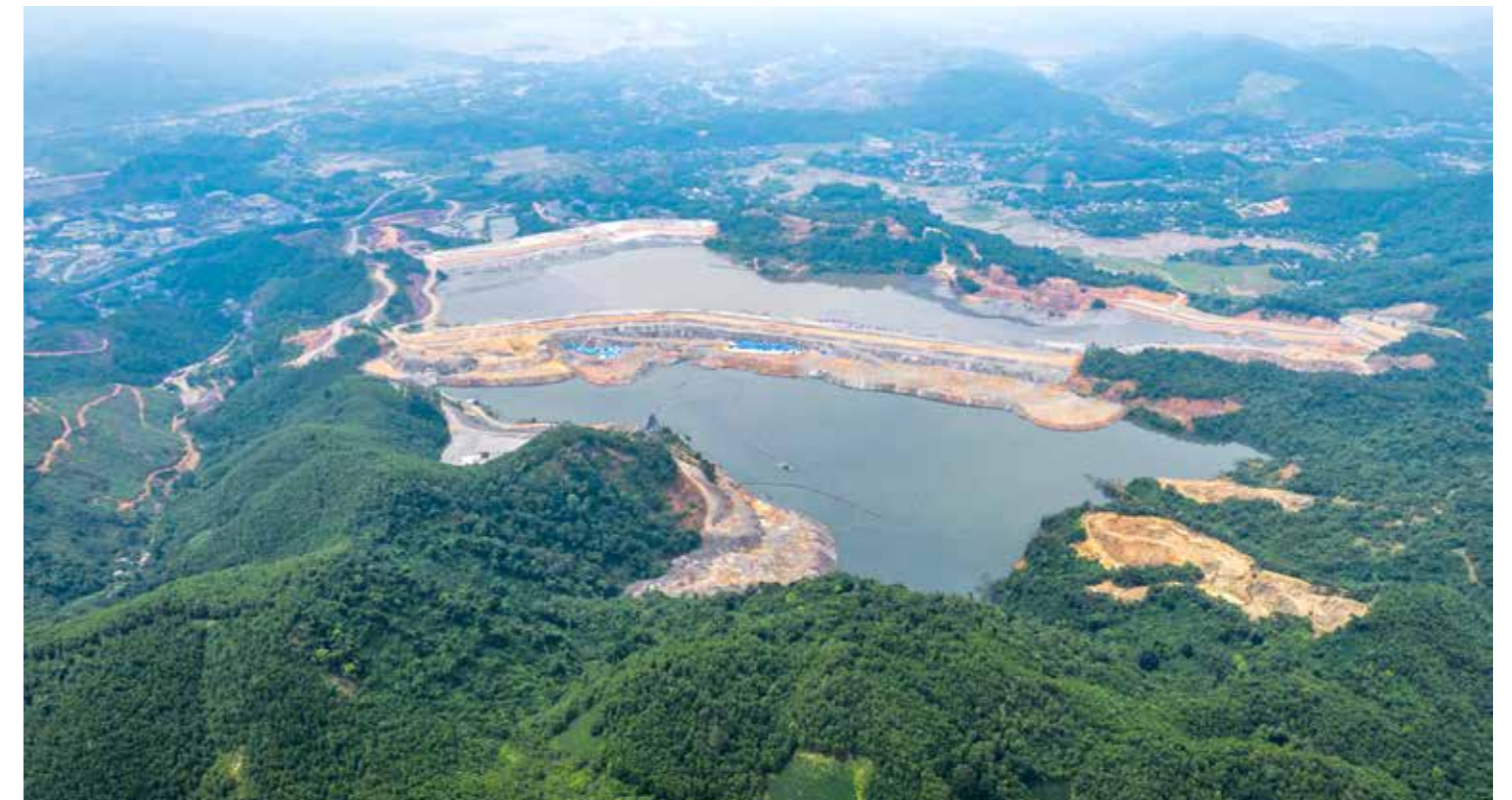
Overview of NPMC tailing dam in Vietnam
