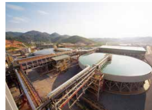
NPMC Processing plant in Vietnam
