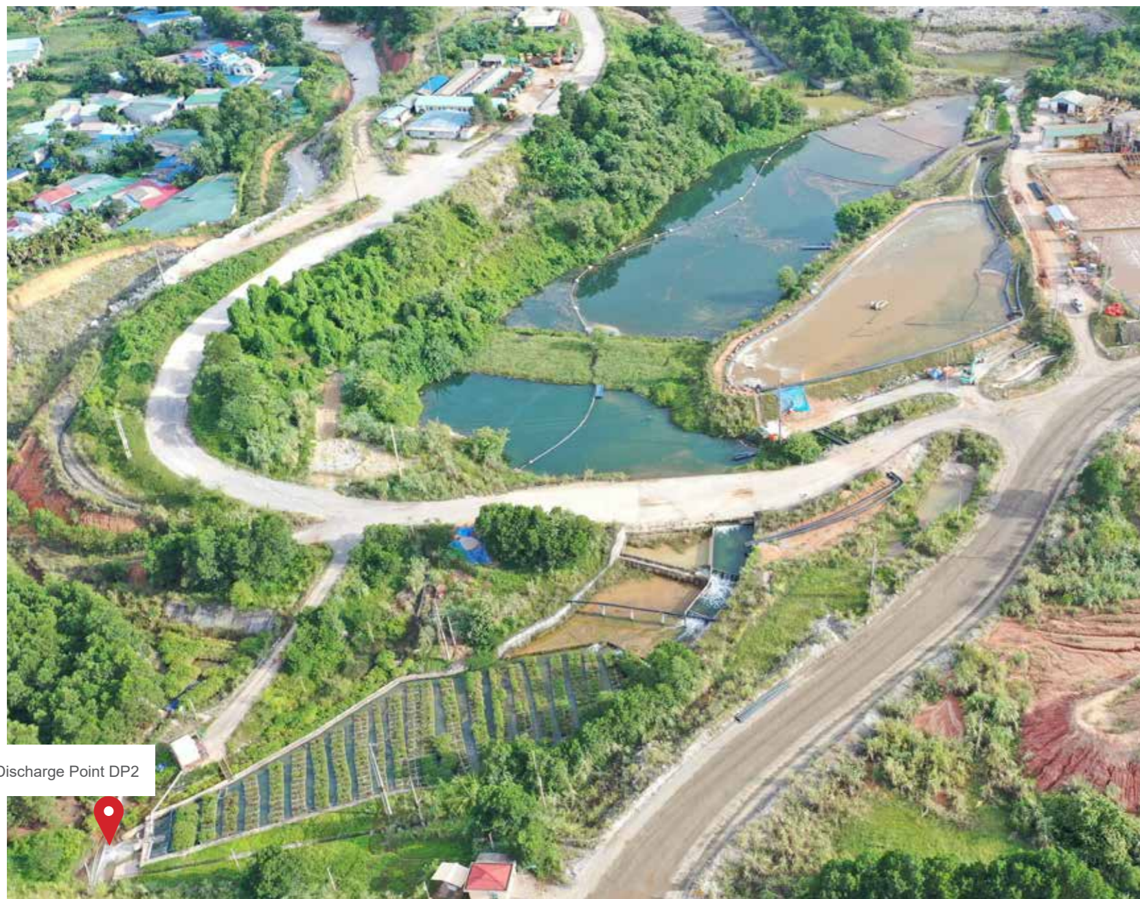
Overview of the wastewater treatment plant and DP2 outlet at NPMC
