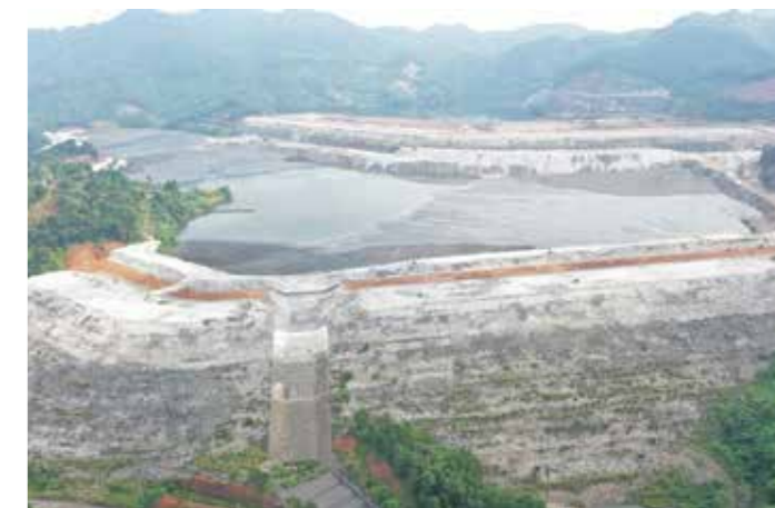
Using waste rock to build dams for OTC and STC ore tailing reservoirs
