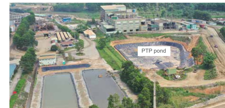
Completed the PTP pond lining
